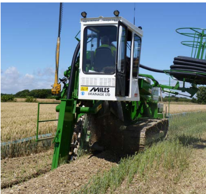
Figure 31. Installing land drains with laser gradient control
