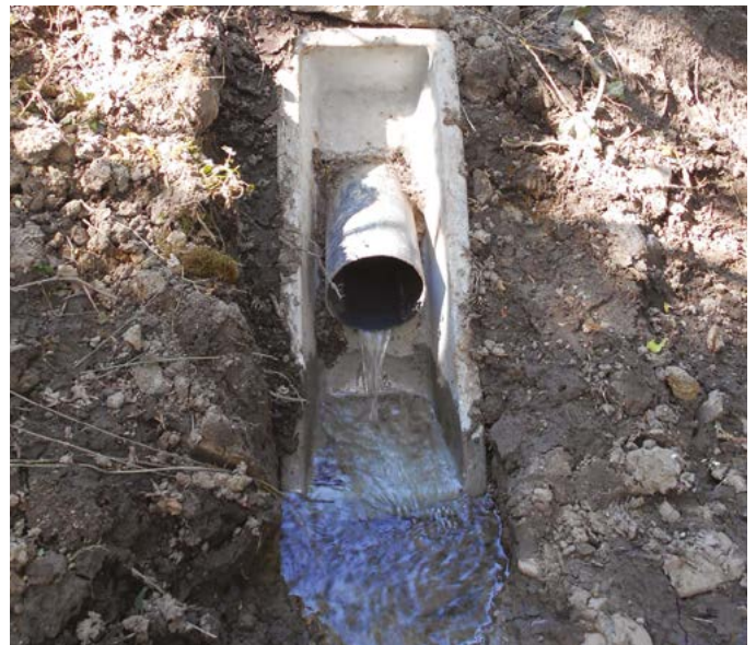
Figure 38. Precast concrete headwall (type K)
