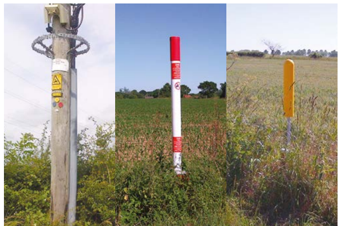
Figure 18. Signs indicating potential underground hazards
