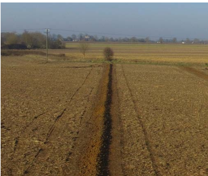
Figure 29. Recently installed drains
