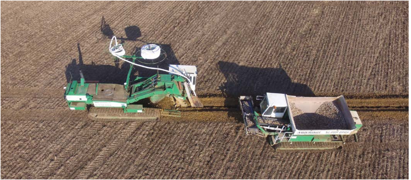
Figure 28. Installing land drains and stone backfill
