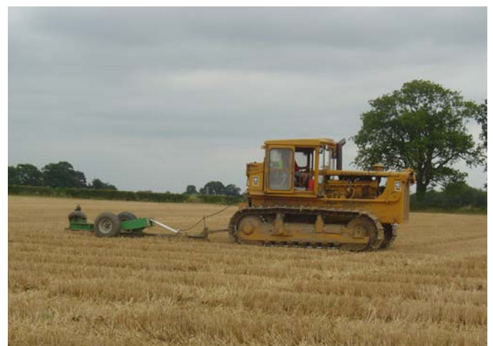
Figure 30. Installing mole drains
