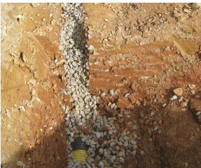
Figure 37. Washed gravel permeable fill over drain
