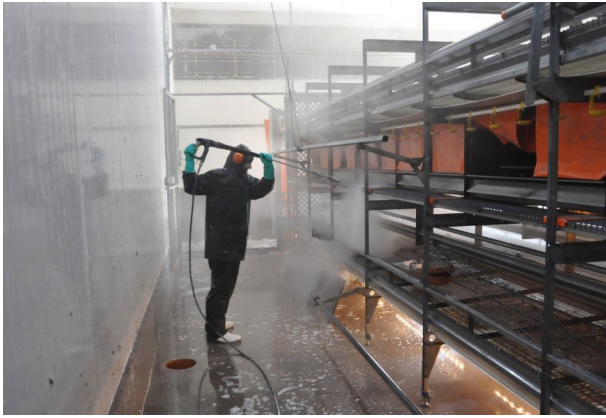
Figure 5: Wet cleaning of aviary housing system
