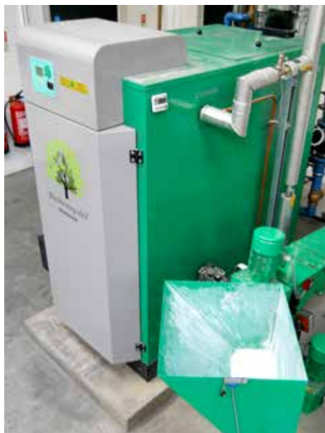
Lime is added to increase the ash melting point of Miscanthus (AFBI)
