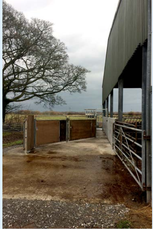
Race with 30 degree angled entrance and solid sides
