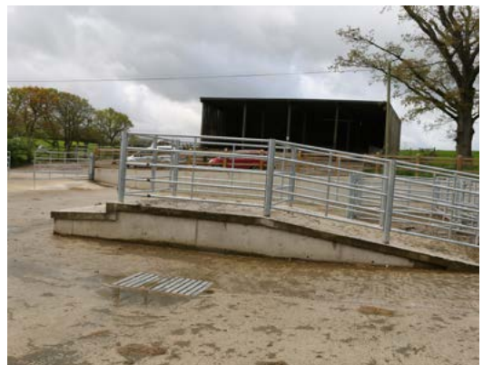
Purpose built loading ramp
